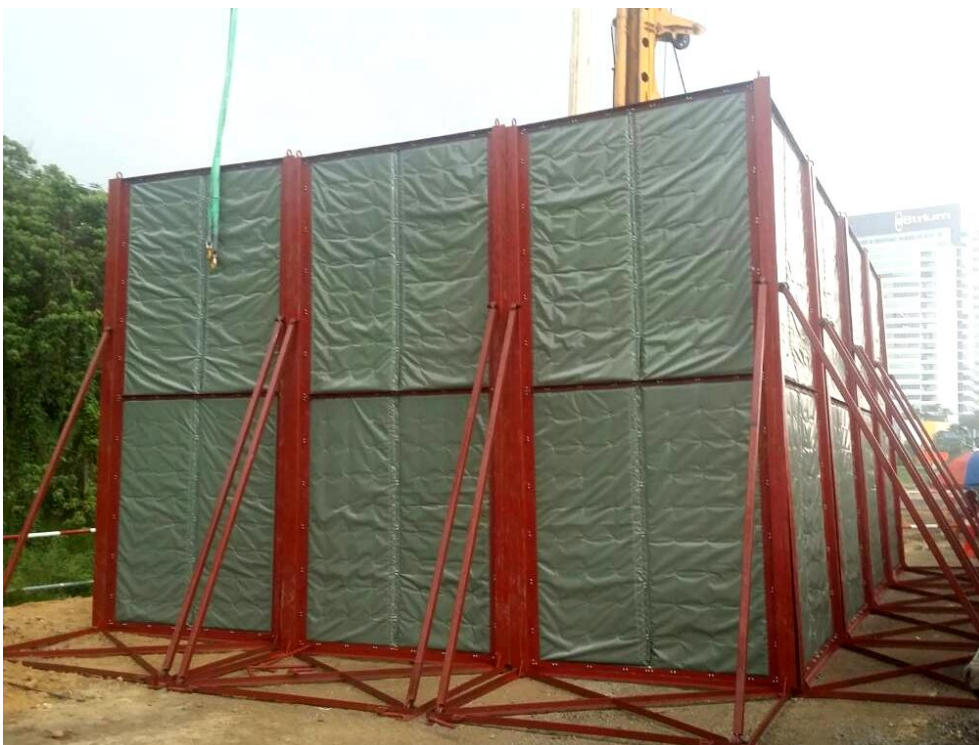
Figure E-12: Movable barrier used for piling noise mitigation
