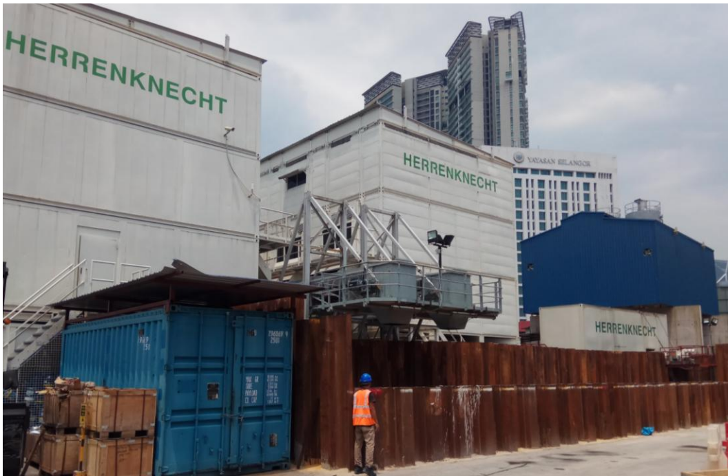
Figure E-15: Full enclosure for slurry treatment plant in Klang Valley MRT construction work site adjacent sensitive receptors
