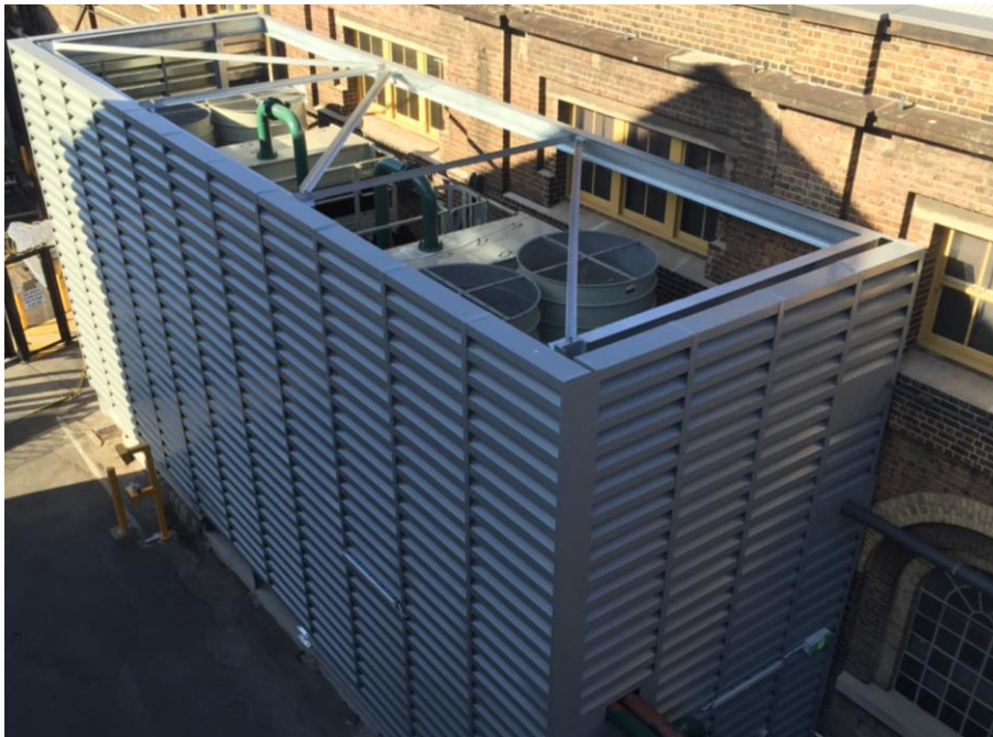
Figure E-23: Acoustic louvers used for cooling towers and chillers noise mitigation
