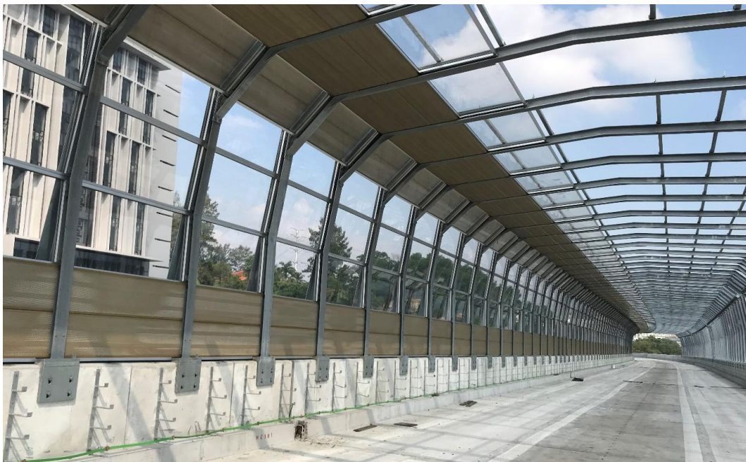
Figure E-19: Semi and partial enclosure for highway and railway noise mitigation.
