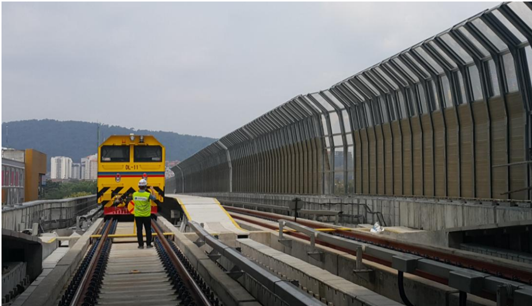
Figure E-7: Metal noise barriers used in railway noise mitigation
