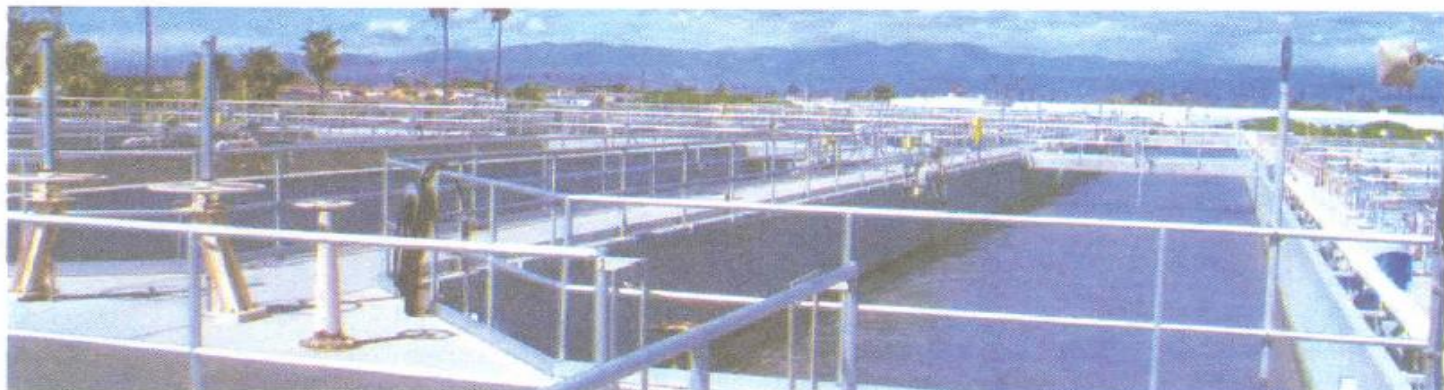
Loji pengolahan air sisa. Wastewater treatment plant.
